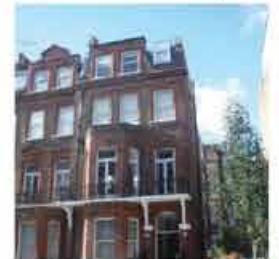
South Kensington. External Repairs and Decoration Project. Contract Value £50,000.
