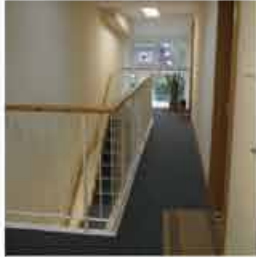
Surrey. Improvement Scheme to Retirement Housing Estate. External, Internal and Landscaping. Contract Value £1.2M.
