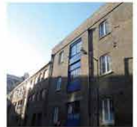
External Renovation of Grade II Listed Building. Residential Converted Victorian Wharf. Contract Value £130,000.
