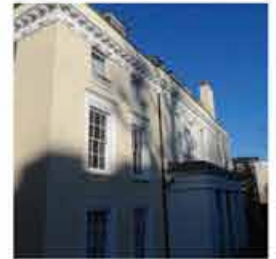
Putney. External and Internal Repairs and Decoration Project. Contract Value £750,000.
