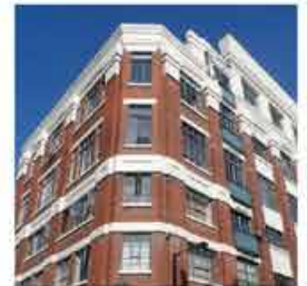
External and Internal Repairs and Decoration Project. Contract Value £150,000.
