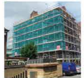
Bethnal Green. External Repairs and Decoration. Converted School Building. Contract Value £110,000.
