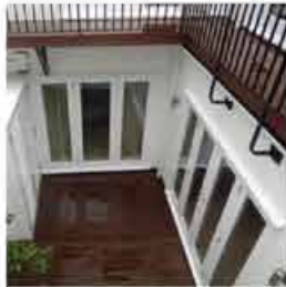
Belgravia, London. Courtyard Refurbishment. Contract Value £35,000.
