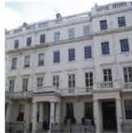
Belgravia, London. External Repairs and Decoration Project. Contract Value £50,000.
