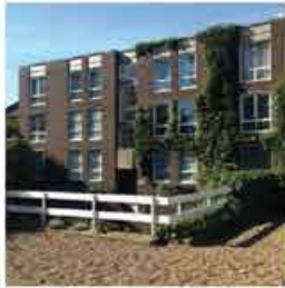
Fulham. External Repairs and Decorations Project. Contract Value £260,000.
