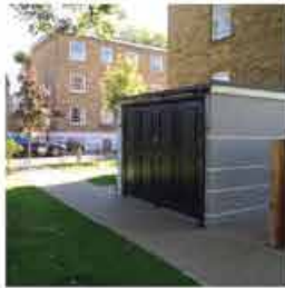
Islington. New Build Bin Stores, Paving and Landscaping. Contract Value £180,000.
