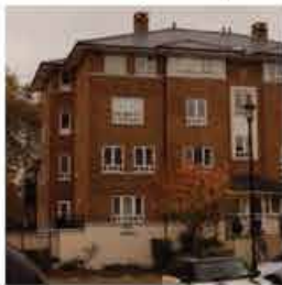
Kingston. Roof Replacement Project. 3 Blocks of Flats. Contract Value £400,000.
