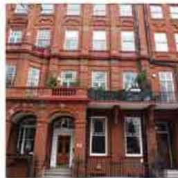
External Decorations and Repairs to a 6 Storey Georgian Style Terraced House. Cadogan Square, London. Contract Value £120,000.
