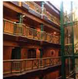
Wapping. Courtyard Refurbishment. Contract Value £120,000.
