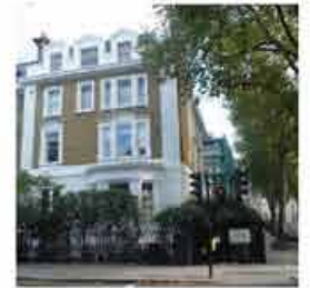
Earls Court. External Repairs and Decoration Project. Contract Value £90,000.
