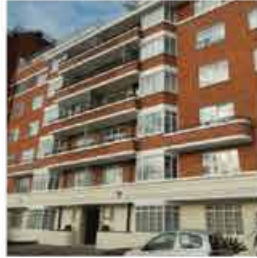
St John's Wood. External Repairs and Decorations Project. Contract Value £600,000.
