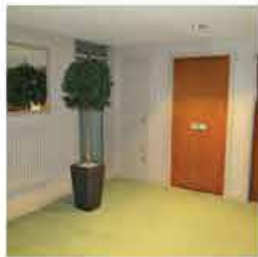
Internal Refurbishment to Communal Areas of Block of Flats. Contract Value £500,000.
