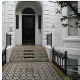
Earls Court. External Repairs and Decoration Project. Contract Value £100,000.
