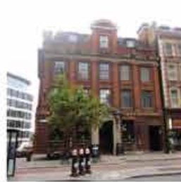
Tower Bridge. External Repairs and Decorations. Contract Value £150,000.
