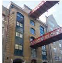
Wapping. External Repairs and Decorations. Wharf Building. Contract Value £120,000.
