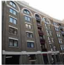
Wapping. Grade II Listed Wharf Building. External Repairs and Decoration. Contract Value £260,000.
