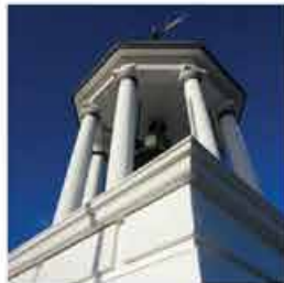
Restoration of Grade II Listed Clock Tower.
