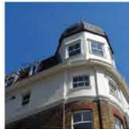
External Repairs and Decoration Project, including Extensive Masonry Repairs. Contract Value £120,000.
